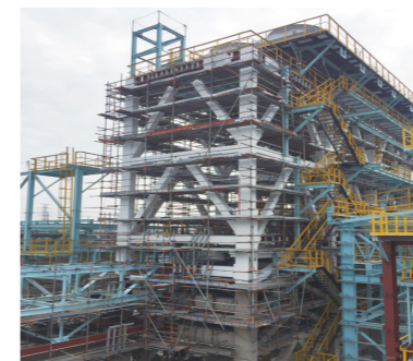
高性能耐火被覆材 / Fireproof cladding (steel column, steel beam, etc.) in petrochemical plant
