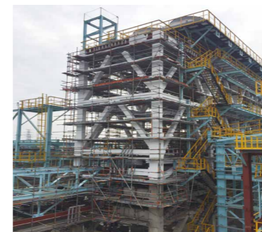
耐火被覆材（鉄骨柱、梁等） / Fireproof cladding (steel column, steel beam, etc.) in petrochemical plant
