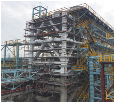
石油化工廠等的防火被覆（鋼柱，鋼樑等） / Fireproof cladding (steel column and steel beam, etc.) in petrochemical plant
